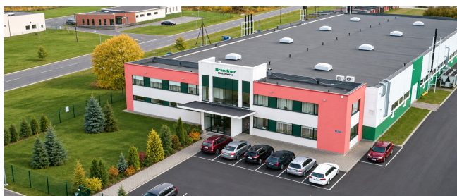
Brandner Electronics OÜ's PCB manufacturing facility in Paide, Estonia.
