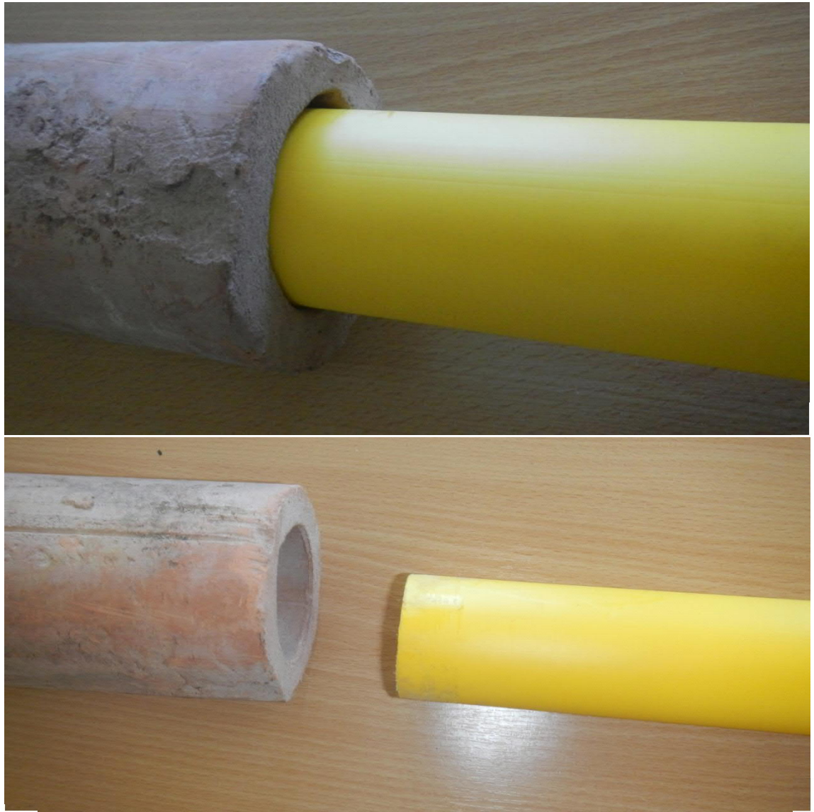
Plastist dreeni paigaldamine savitorusse DN50
