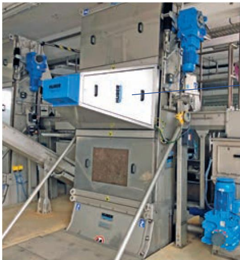
Figure 1: HUBER Safety Vision installed on a HUBER Multi-Rake Bar Screen RakeMax®.
