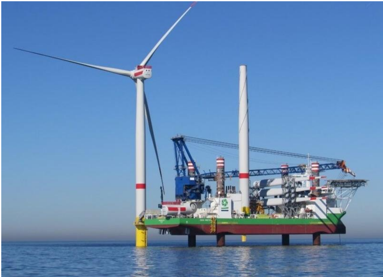
Figure 9. Installation of wind turbines by a jack-up vessel. Source: COWI
